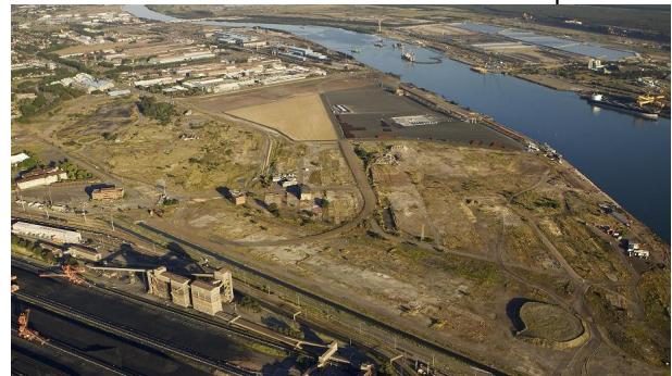
AERIAL VIEW AFTER STAGE 1 REMEDIATION
