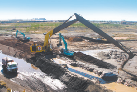
The $20M underground barrier wall was constructed using the world's largest long arm excavator, specially imported from the USA.
