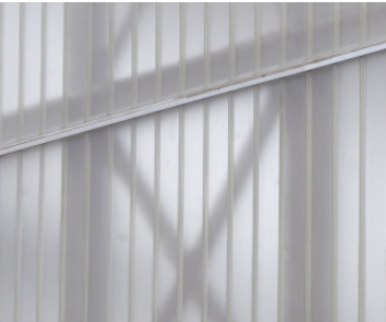
TRANSLUCENT GLASS UPPER FACADE WITH EXPRESSED STRUCTURE BEHIND
