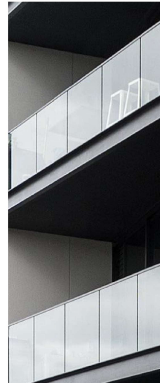
Bronze coloured handrail + Frameless glass balustrades
