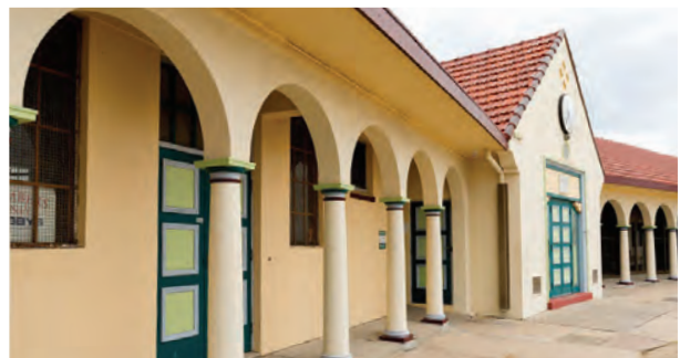
Nobby's Beach Pavilion refurbishment; Funded through the Newcastle Port Community Contribution Fund
