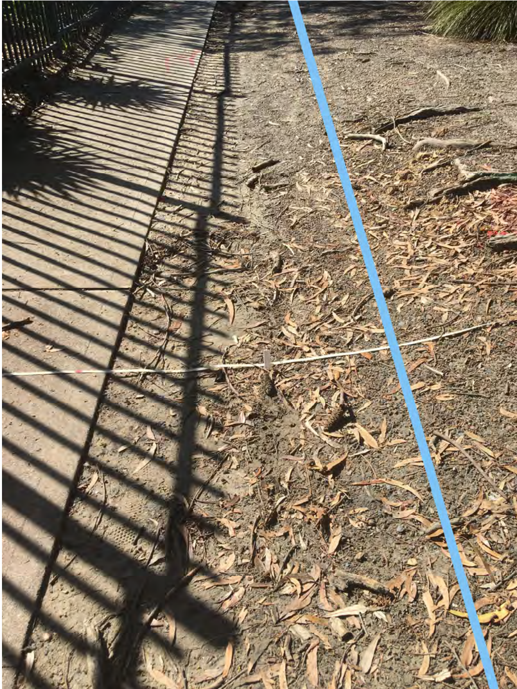
Figure 2. The blue line indicates the approximate edge of the proposed shared pathway. Note severed roots to the right of the blue line.
