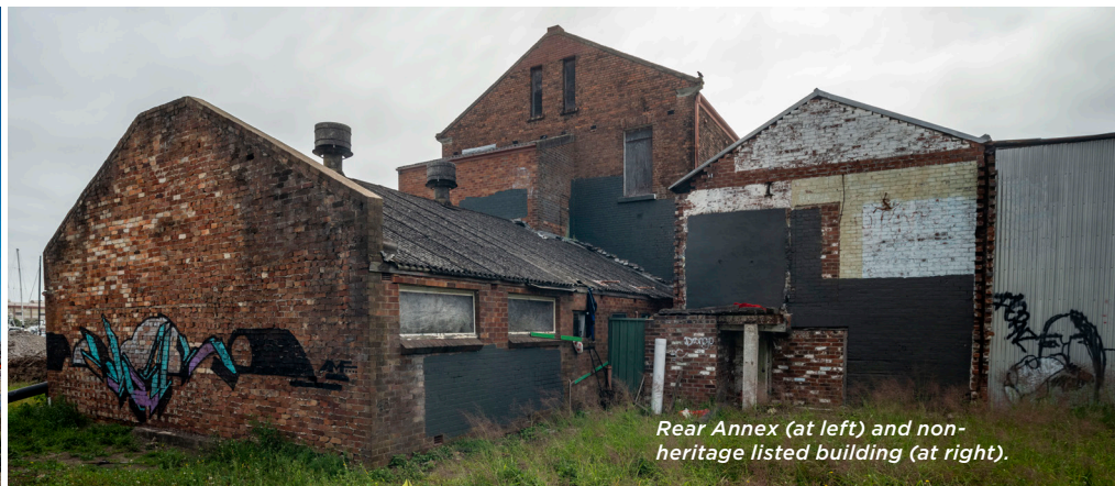
Current state of former Wickham School of Arts Building.
