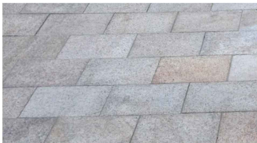
P1- in Tier 1 paving Material: diamond gold granite unit paver Size: 600x300x40, 600X600X40 400x300x40mm Finish: exfoliated finish/ bush hammered finish Pattern: staggered stretcher bond
