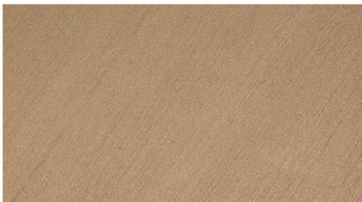
P3- in Tier 2 paving Node base paving: insitu concrete/ coloured concrete solutions (CCS) : Colour/Size: kalgoorlie full body oxide colour 20mm river gravel Finish: honed
