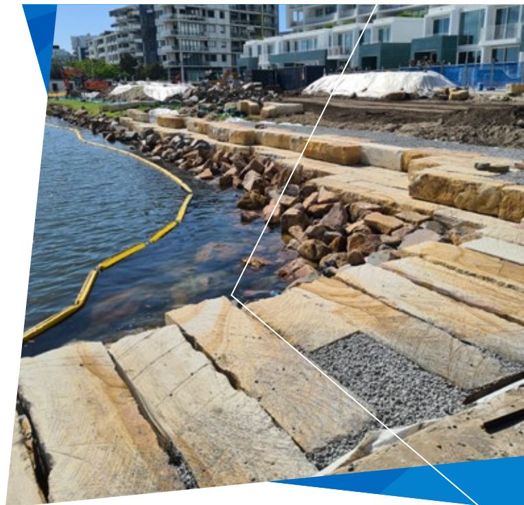
Installation of sandstone seating will offer residents and visitors a new way to enjoy the Honeysuckle foreshore.
