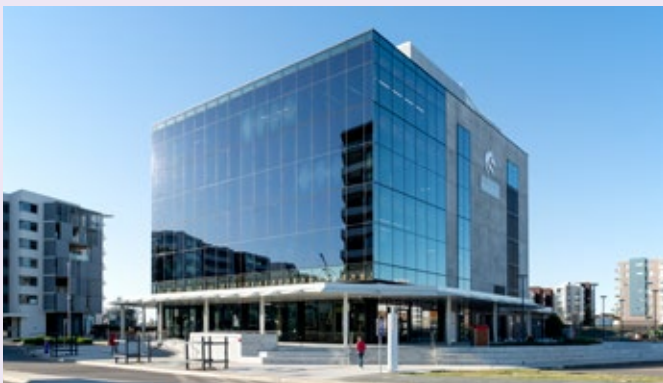
UoN's Q Building received the first 6 Star energy rating in regional NSW.
