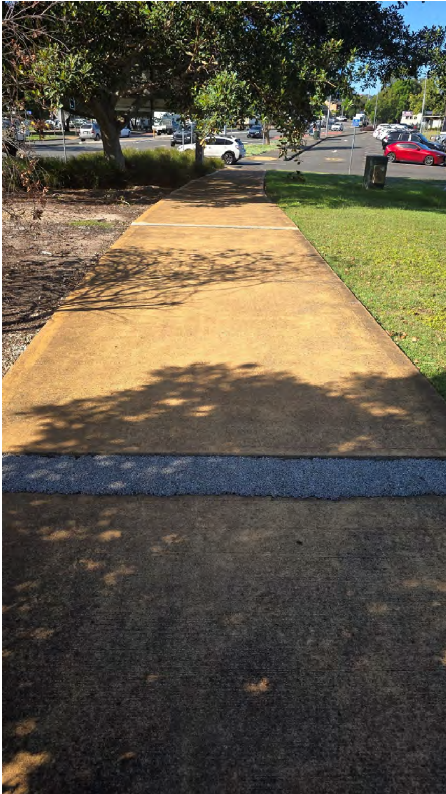
Plate 2 - Tree 6 on the left and the proximity of the roots to the current path. Grinding and ramping are already used to manage risks. landscape design should address this problem.
