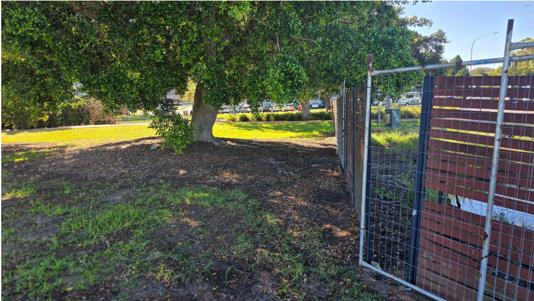
Plate 3 - Tree 5 looking east. The current temporary fence is sufficient to protect this tree and the previous excavation on the site. The tree has a large NRZ area however no further encroachment to that present will occur.
